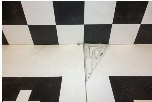
Finding a line perpendicular to the wall
